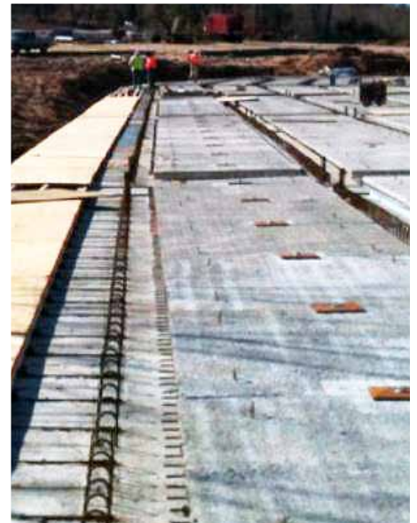
JW Payne crew installing bridge overhang
